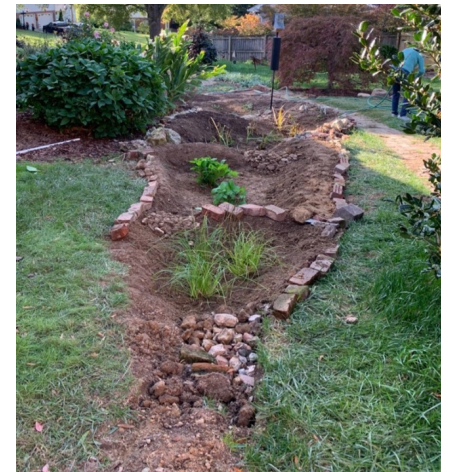
Last fall, WaterWays staff installed a tiered rain garden at a East Brainerd residents home.
