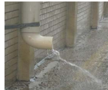
This downspout connects to the roof gutter.
