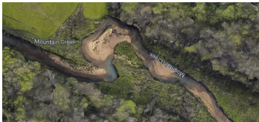
Preliminary design plans for the Mountain Creek Church of Christ restoration project (top photo) vs current stream channel (bottom photo).
